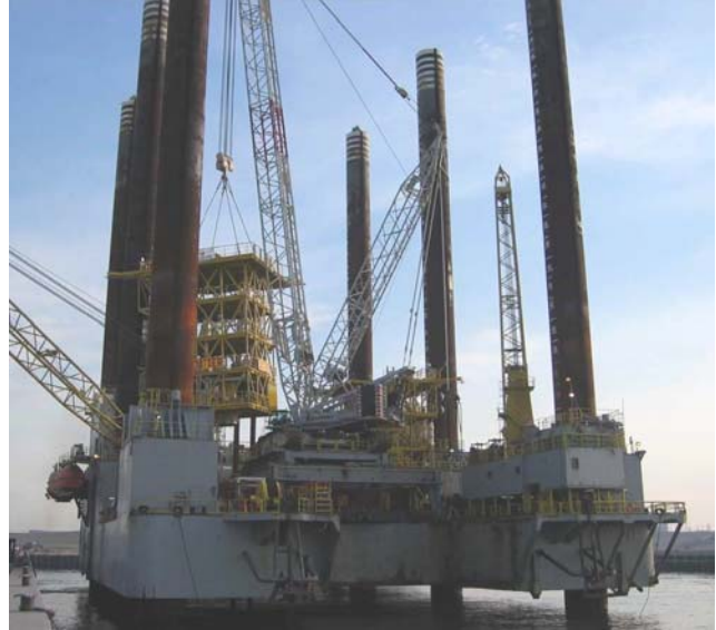
Fig 4. Load out platform
